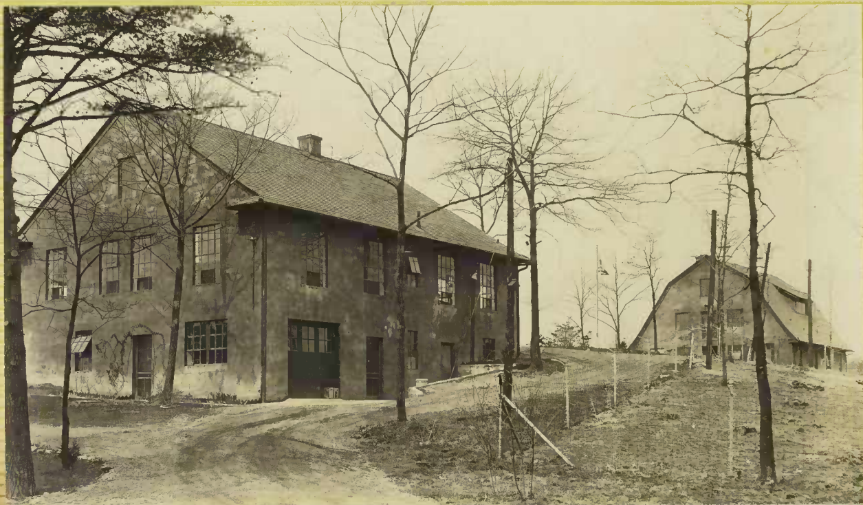
Laboratory on left; animal and feed-storage barn on right.
