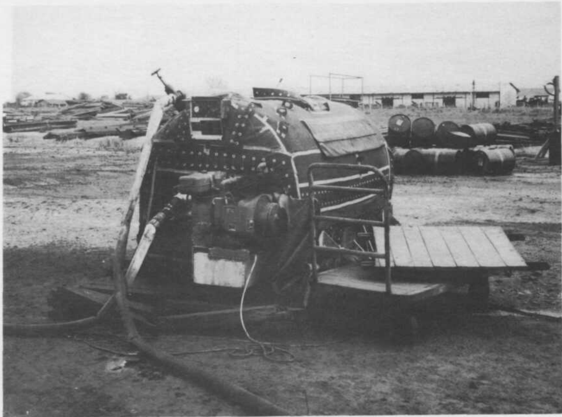
Figure 13. Hour Glass Tank and Pump (Insulated)
